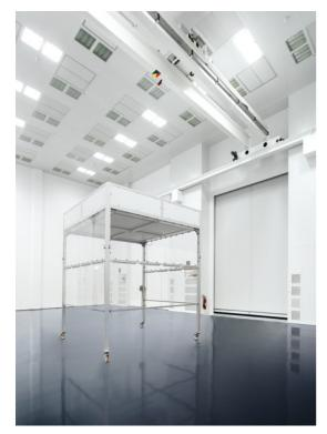
Air can easily overcome barriers and can, hence, not be locked out. With the air management system it is possible to precisely control pressures in the clean room and adjoining areas and to isolate rooms with particularly critical requirements of air cleanliness from those with less critical requirements.
